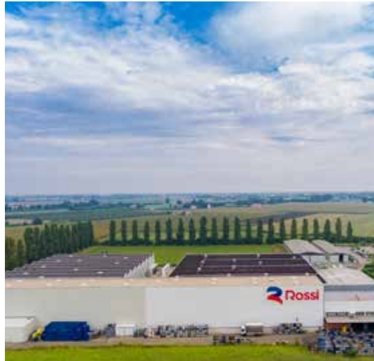
High precision manufacturing facility Ganaceto (Modena) - Italy
