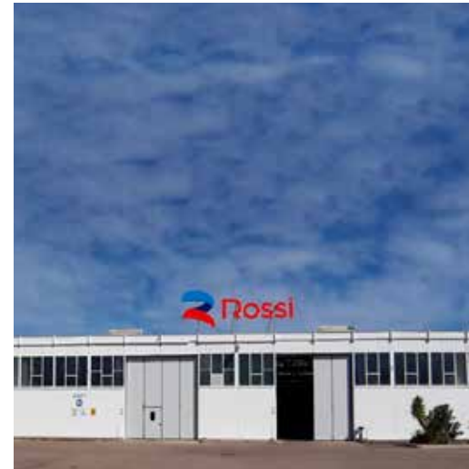
Planetary Division facilities Lecce - Italy
